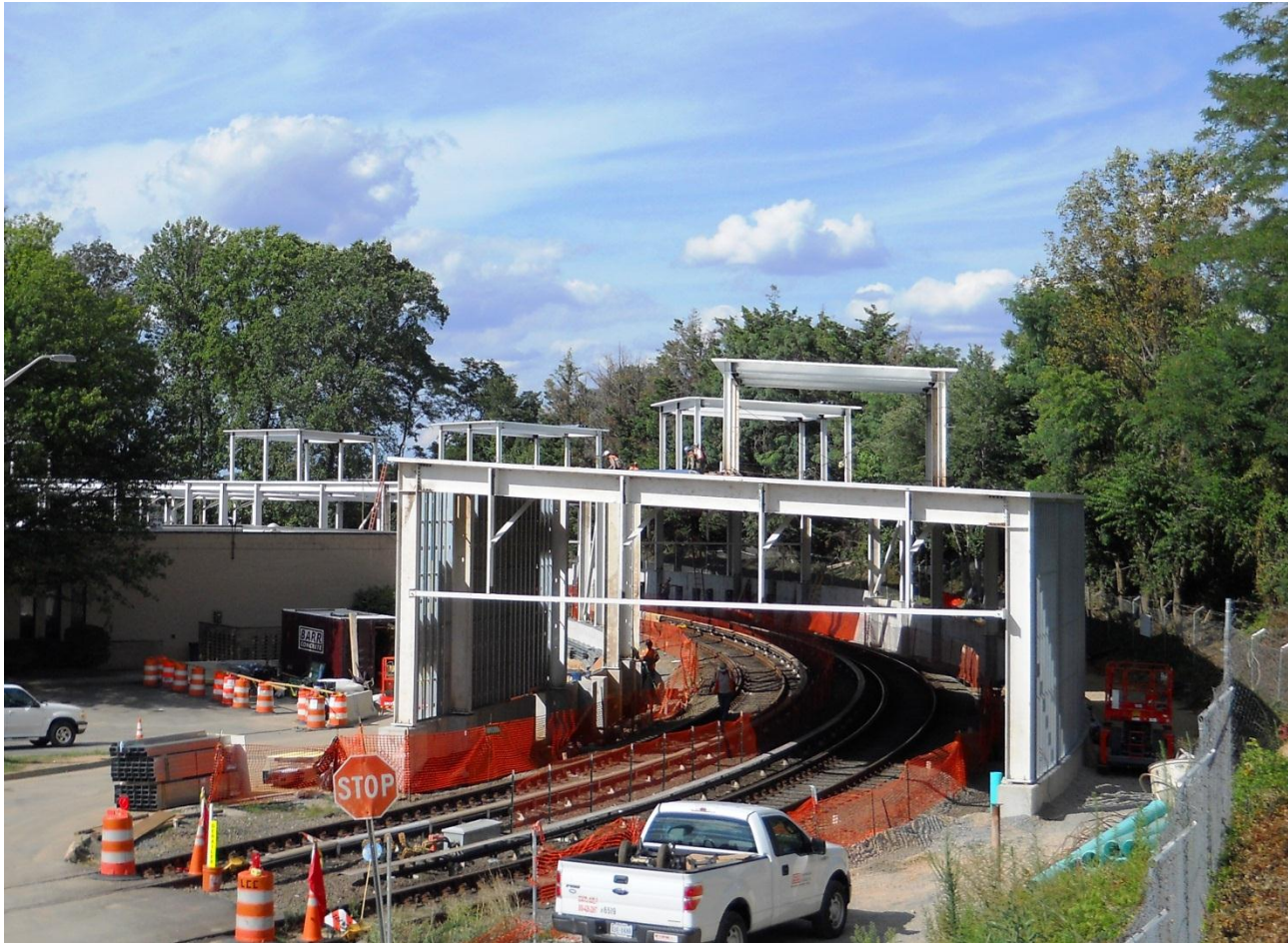
West Falls Church yard sound cover box. Structural steel framing of the south portal to the loop track sound cover box. Photo courtesy Stephen Barna, Dulles Corridor Metrorail Project (DCMP).
