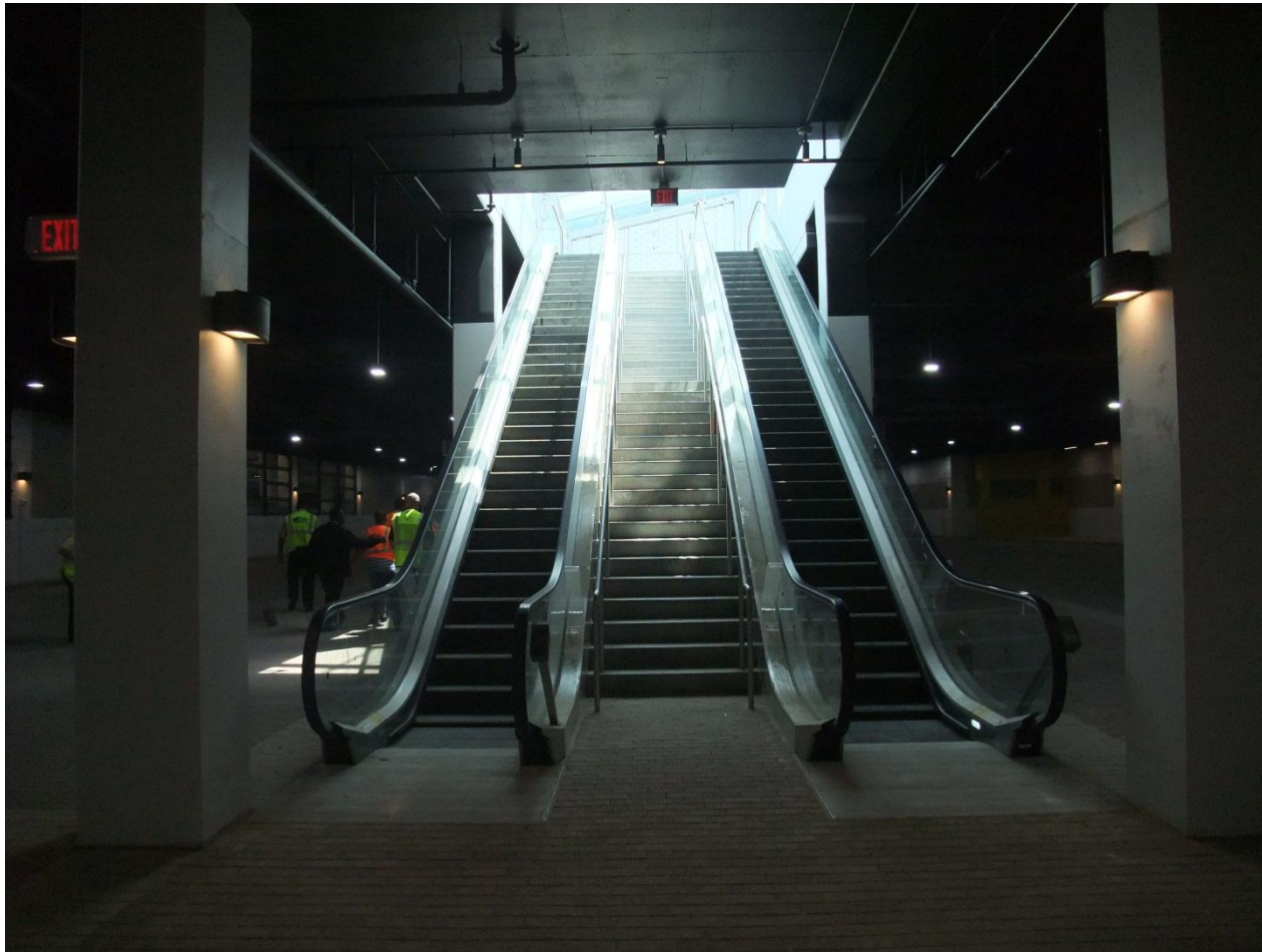
Escalators and stair case connecting the bus platform with the pedestrian plaza. Photo courtesy Ellen Kamilakis, FCDOT.
