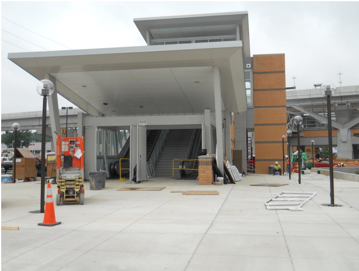
Spring Hill Station north entrance pavilion – window/curtain wall glazing, entrance gates, plaza sidewalk, and site lighting are complete. Photo courtesy Stephen Barna, DCMP.
