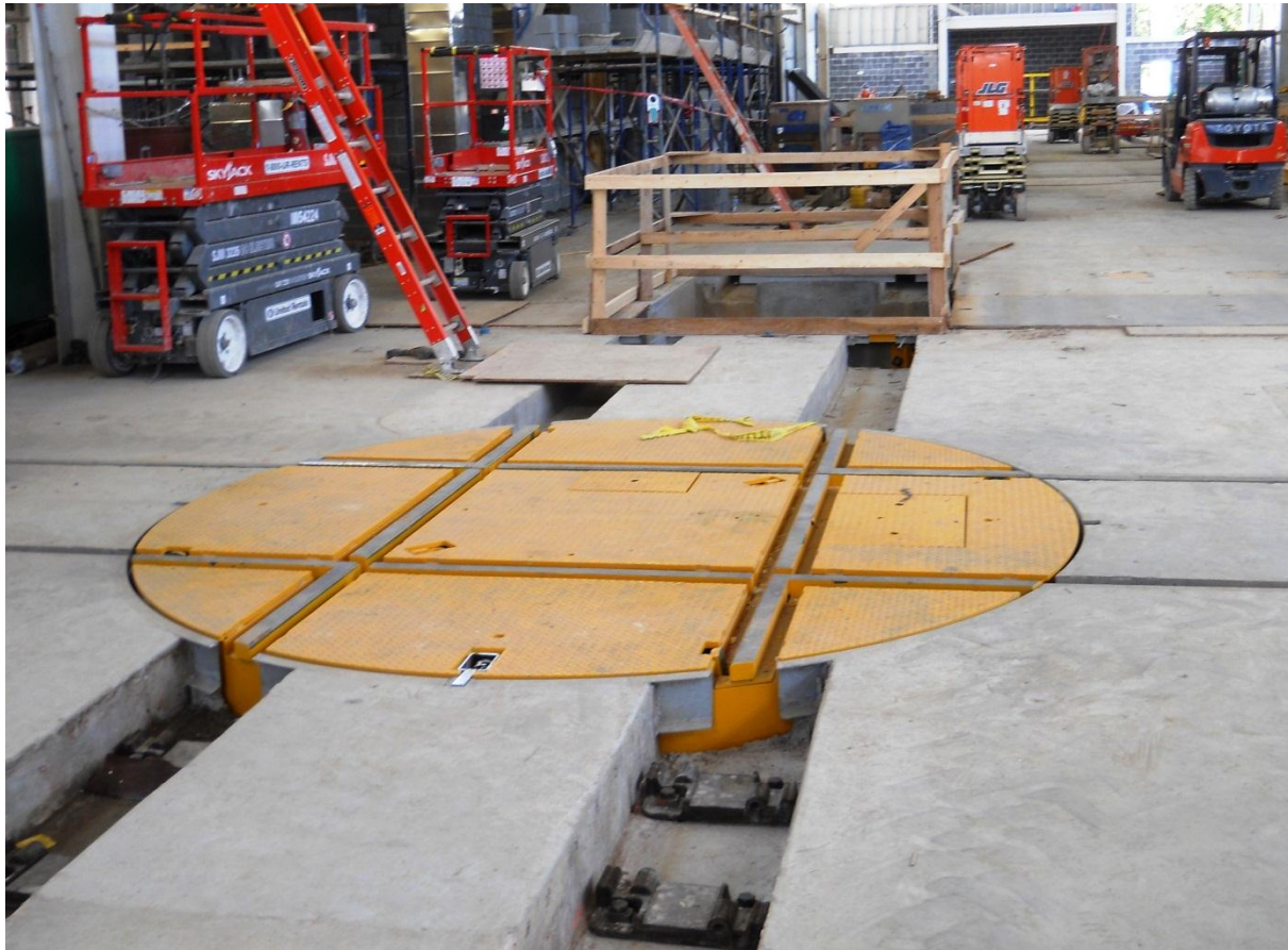
West Falls Church yard service & inspection Building. Turn tables in the shop floor have been installed. Photo courtesy Stephen Barna, DCMP.
