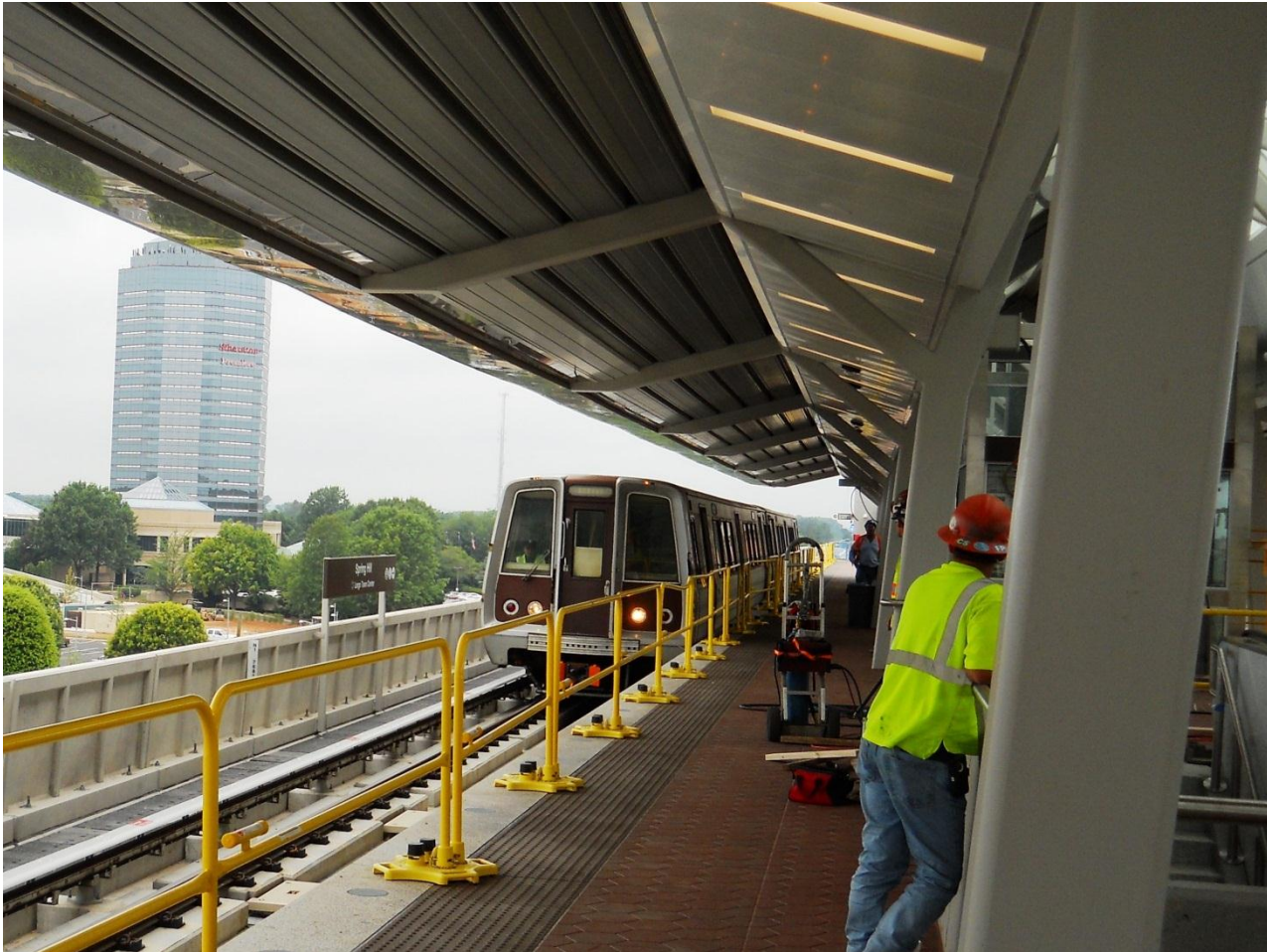
Spring Hill Station platform – WMATA test train passing through the station on the inbound track during dynamic testing. Photo courtesy Stephen Barna, DCMP.
