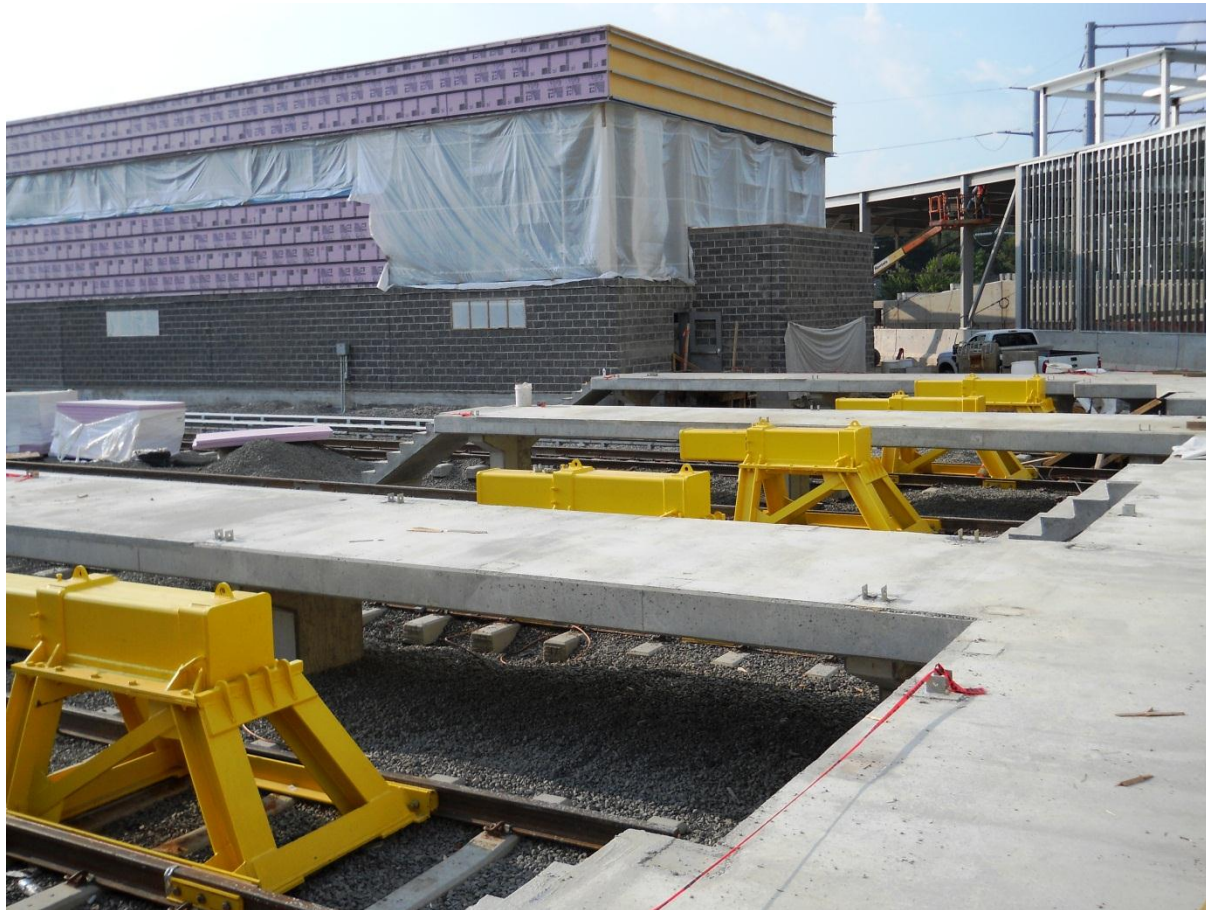
WFC yard - train access platforms are complete except for handrails; new storage track bumpers are installed; the Service & Inspection Building and sound cover box nearing completion. Photo courtesy Stephen Barna, DCMP.
