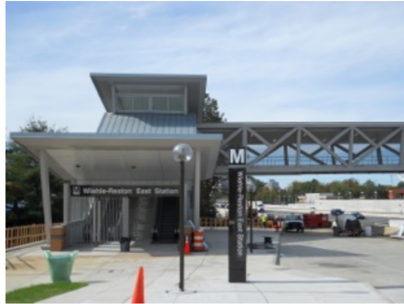
Wiehle-Reston East Station south pedestrian pavilion with completed Metro entrance pylon. Completed Wiehle south bus lane/bays is to the right of the Metro pylon. Photo courtesy Stephen Barna, DCMP.
