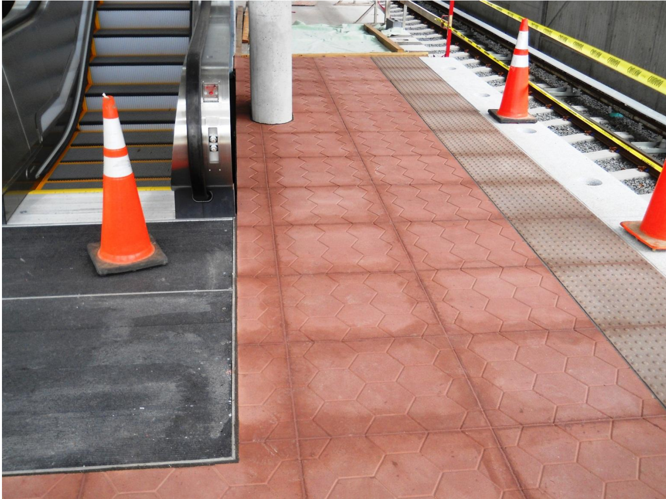
Wiehle Station. Concrete “tile like” platform surface. Photo courtesy Stephen Barna, DCMP.
