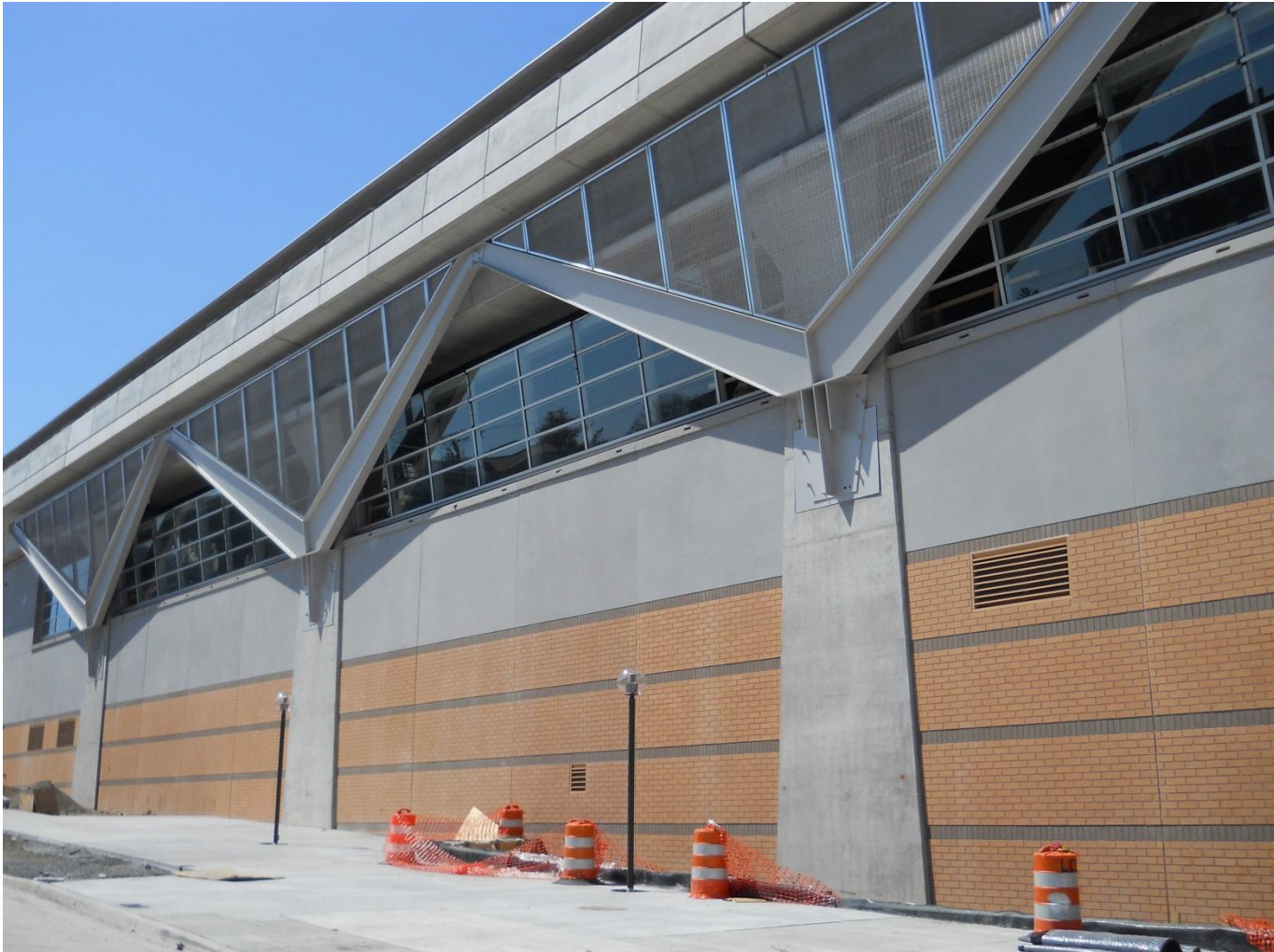
McLean Station looking north. The station curtain wall and “V” framing nearing completion. Photo courtesy Stephen Barna, DCMP.
