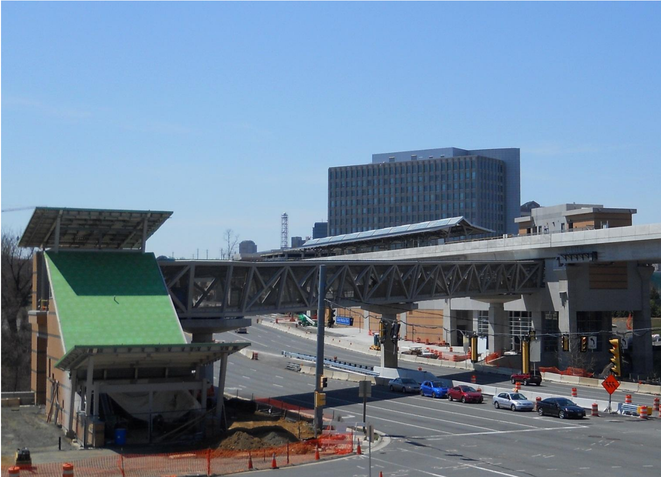
McLean Station looking west. Installation of the pedestrian bridge wire mesh nearing completion. Photo courtesy Stephen Barna, DCMP.
