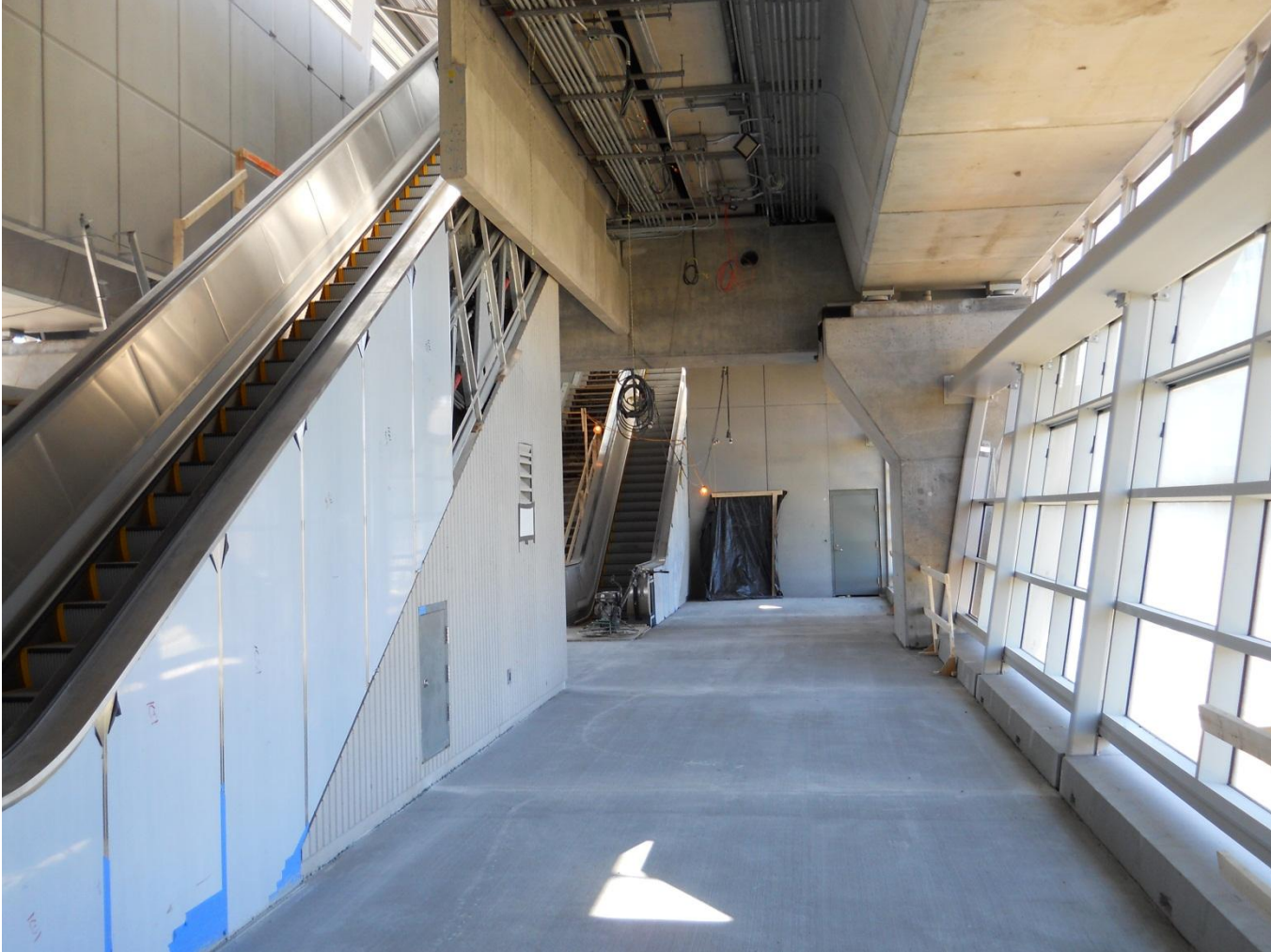
McLean Station mezzanine to platform escalators and curtain wall nearing completion. Photo courtesy Stephen Barna, DCMP.
