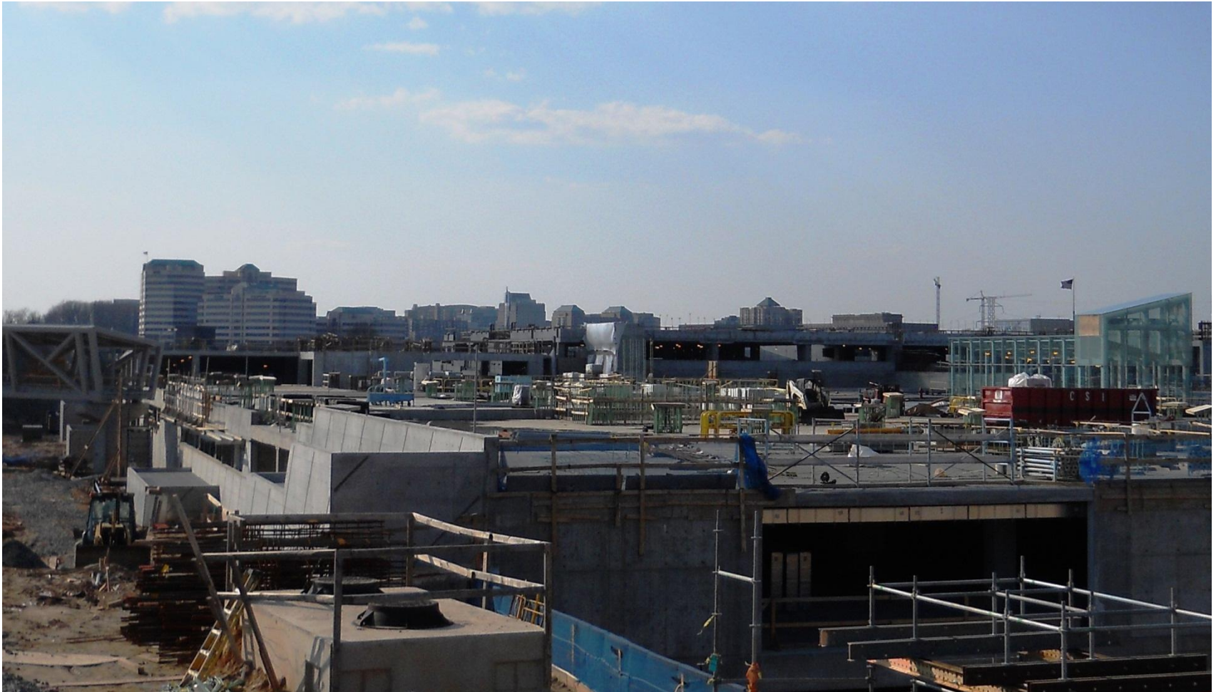
Wiehle Station looking west, north side pedestrian plaza. Steel-framed glass structure enclosing the elevators and escalators to the bus plaza below. Photo courtesy Stephen Barna, DCMP.
