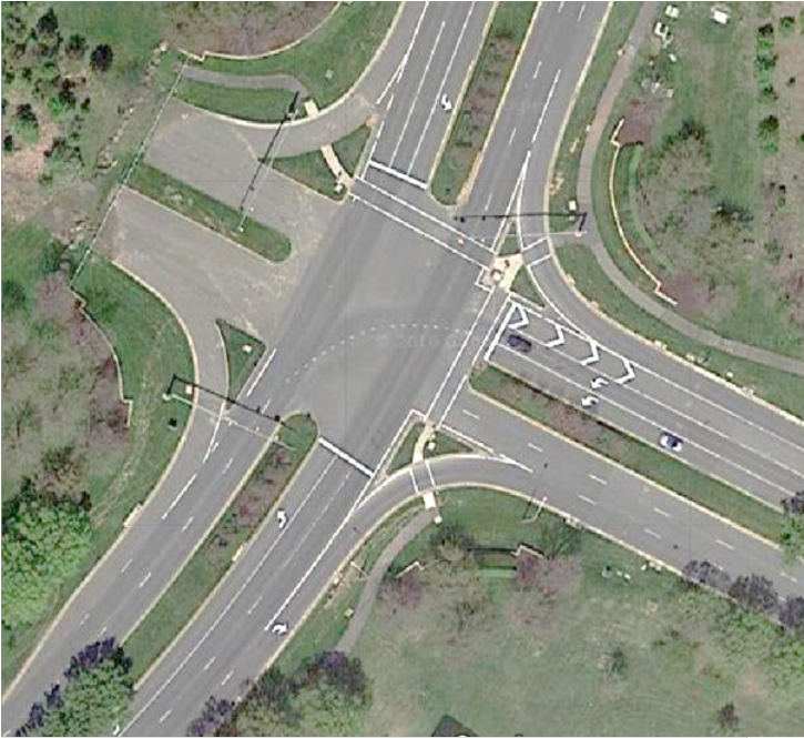
Existing Westfields and Newbrook Intersection
