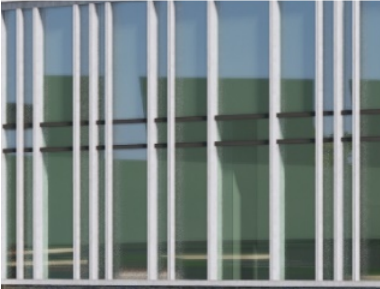
VERTICAL MULLION WITH SNAP-ON COVER EXTENSIONS
