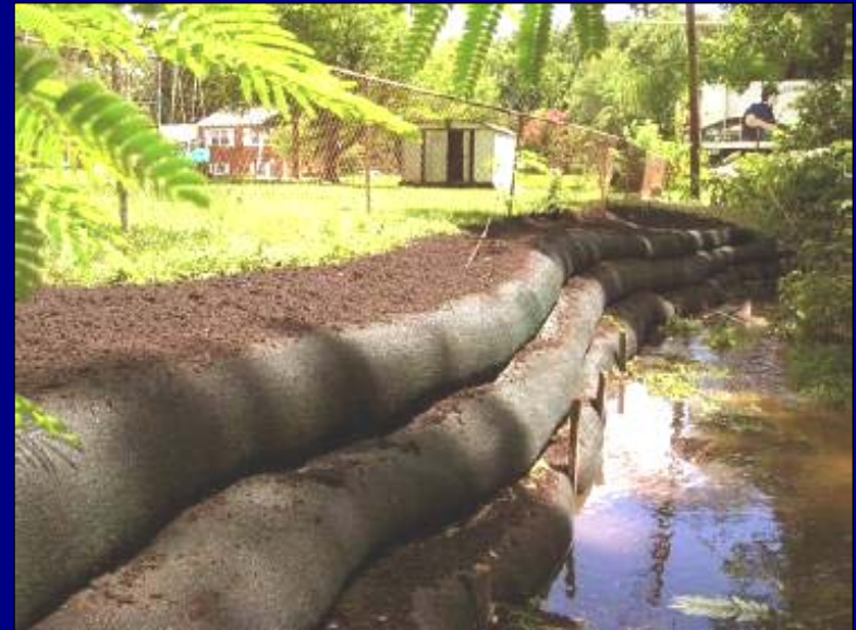
Bioengineered using Filtrex along banks
