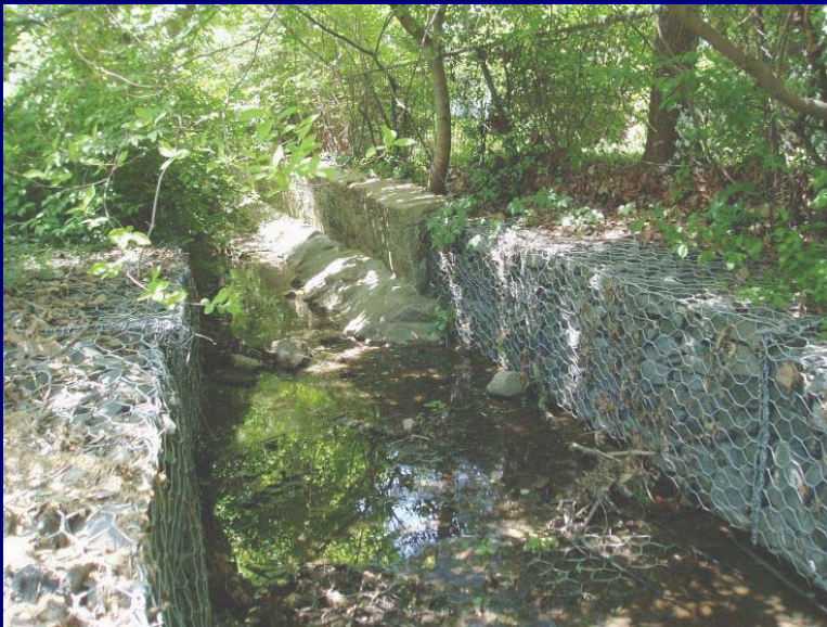
Not bioengineered using gabion
