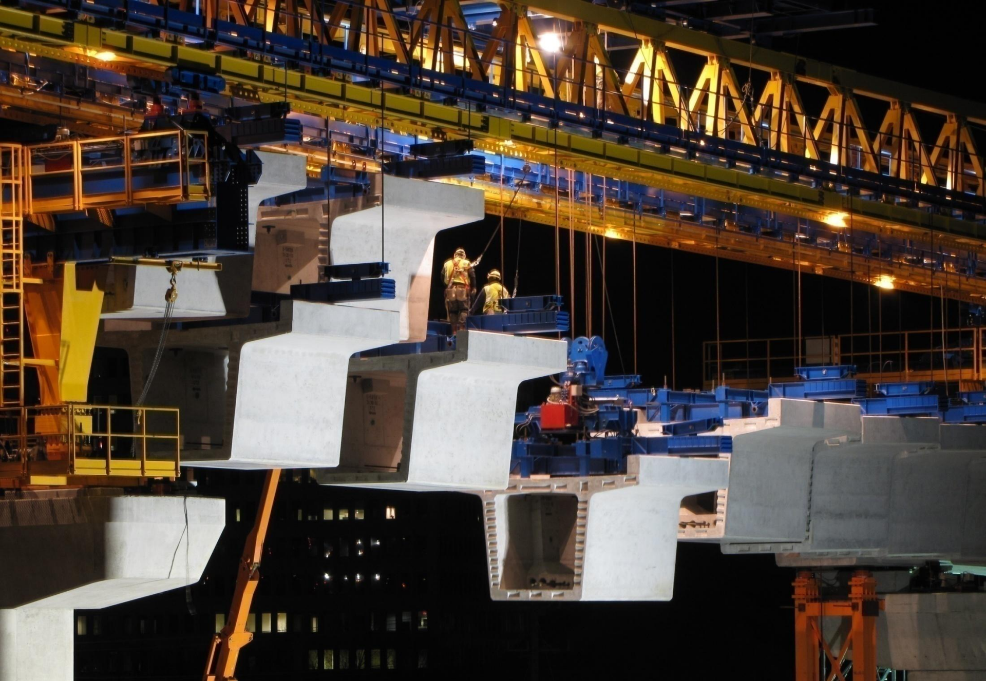
Concrete segments being erected for spans
