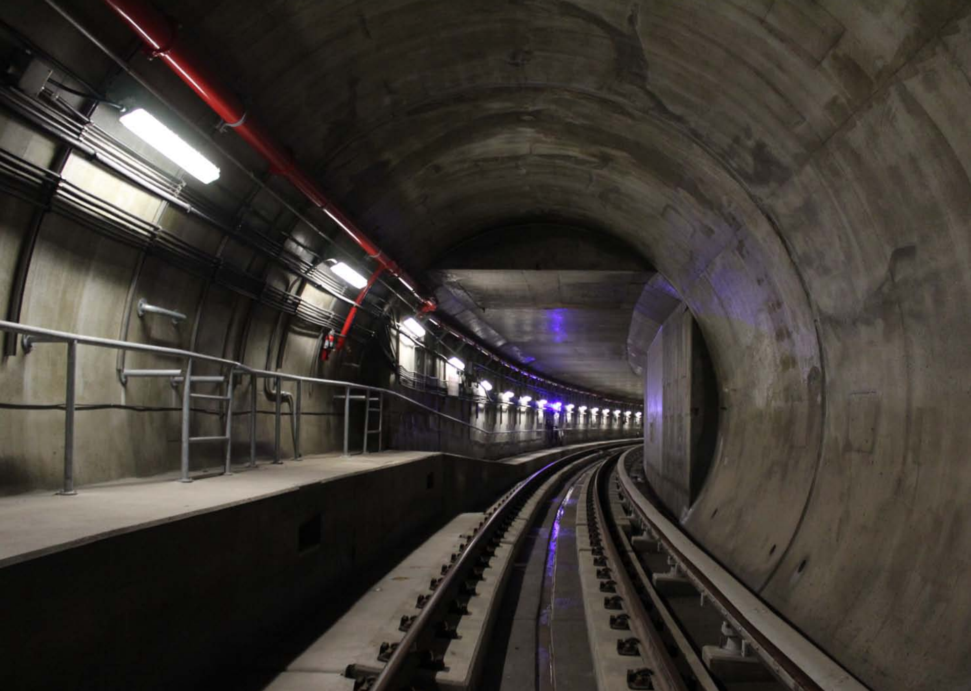
Tunnel below Route 123 and Route 7
