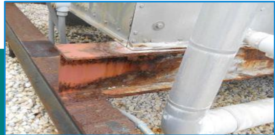
Deteriorating Mechanical Unit Supports
