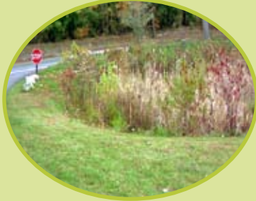
Constructed Stormwater Wetlands
